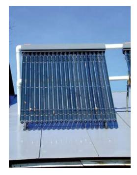
An evacuated tube collector provides hot water to a Vermont farm home. Courtesy of DOE/ NREL; Credit: Alan Ford
